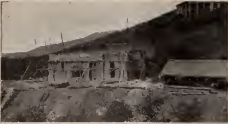
Tooker Memorial Chapel, Hangchow, China, in process of construction.
